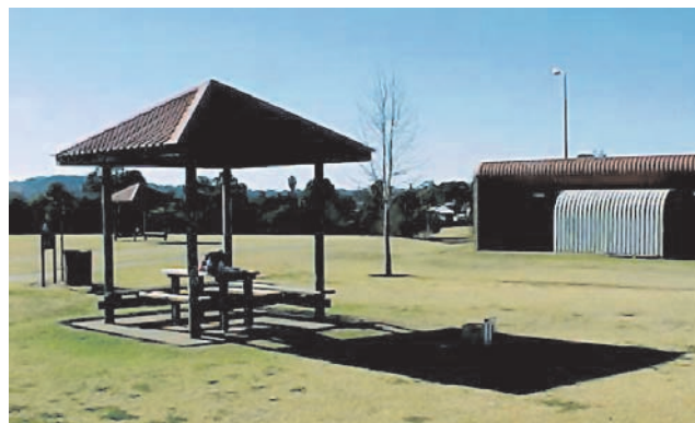
The shade provided by the structure is not over the table and seats.♦
