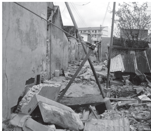
1 Tsunami damage in Kandholhudoo on the Raa atoll
