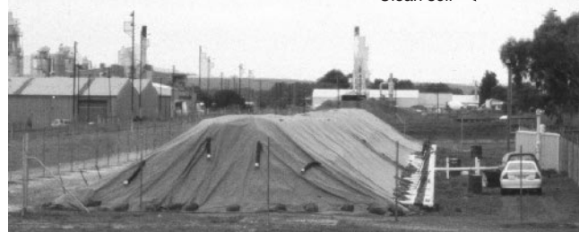
Biopile for the remediation of diesel-contaminated soil from an old railway yard. Moist soil is stockpiled, and endogenous bacteria are stimulated to degrade diesel hydrocarbons by addition of inorganic nutrients.
