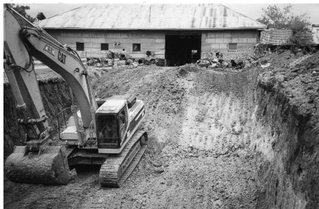
A contaminated, abandoned mineral processing site. A containment cell is being constructed on site for depositing waste.
