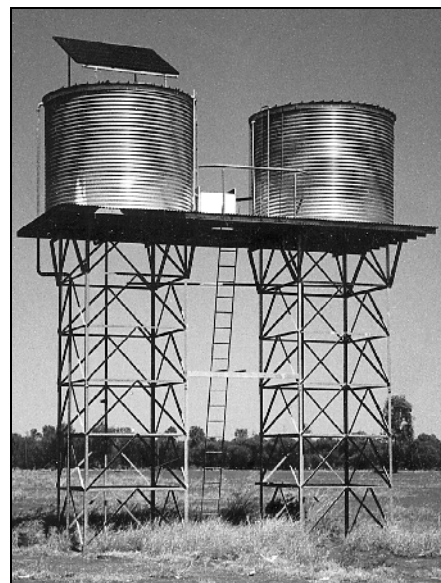
These tanks are fitted with solar-powered reverse-osmosis filter systems to reduce levels of dissolved solids and render the water palatable.
